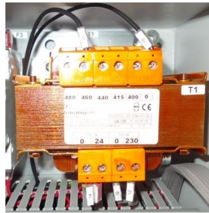
Connection to power supply 460V-3-60Hz
