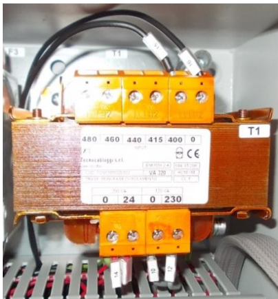
Connection to power supply 400V-3-50Hz
